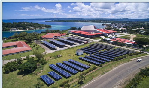
Solar Solutions for the Government; Parliament building complex, Port Vila Vanuatu; Source: https://www.sunergisgroup.com/parliament-house-vanuatu
